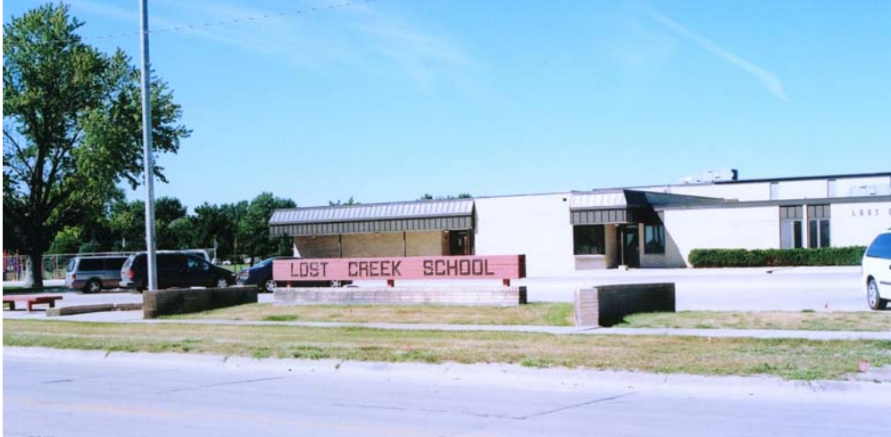
Lost Creek Elementary School
